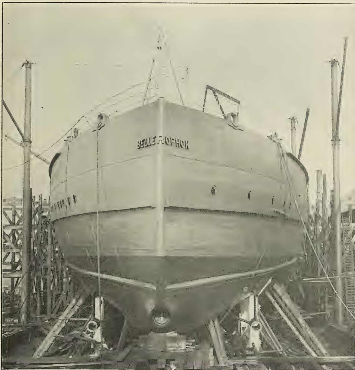
STERN OF THE BELLEROPHON BEFORE LAUNCHING, SHOWING STERN TORPEDO TUBE AND TWO OF THE PROPELLER STRUTS.
